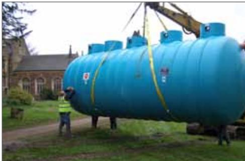
Consideration in the final specification of the product was given to the need of the final effluent to be of a high standard to meet the required low Ammonia & BOD levels. The estate is surrounded by lakes with high levels of fish and wildlife. Marsh Industries was chosen and provided detailed design schedules to the Consultant Engineers. Due to the variations in daily loadings a Marsh Ultra Polylok 135PE was specified.
